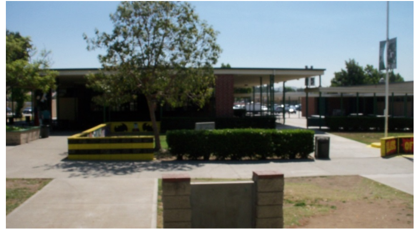
Former Cafeteria Building
