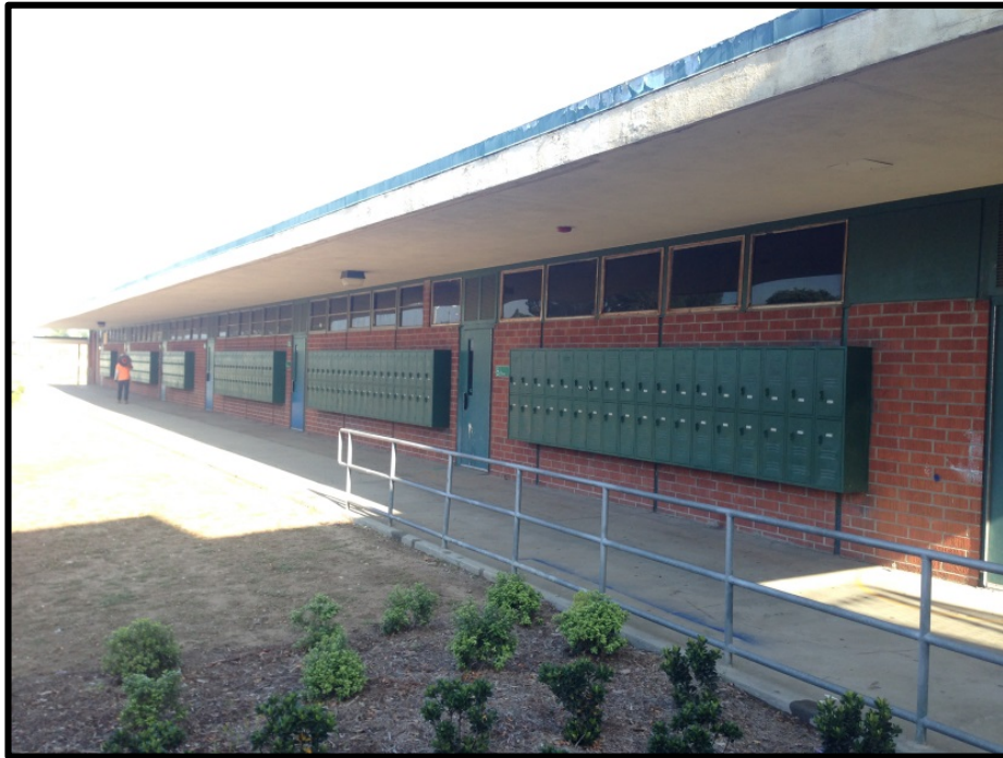
Replacement of Building F
