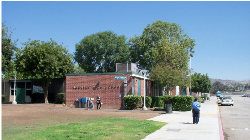
Former Admin. Building – South Elevation
